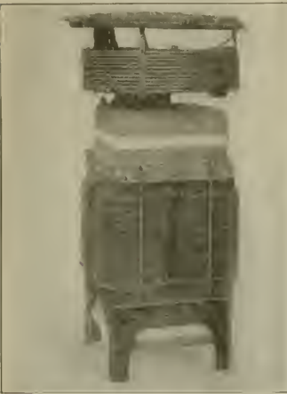
FIG. 4. DRYING TRANSFORMER.
